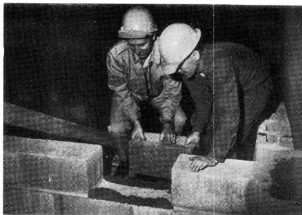
Captain W. K. Martin assists in laying the last block in the handball courts.
